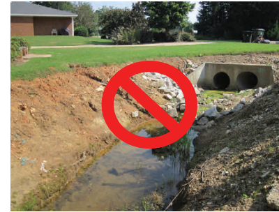
No Stream Buffer!
